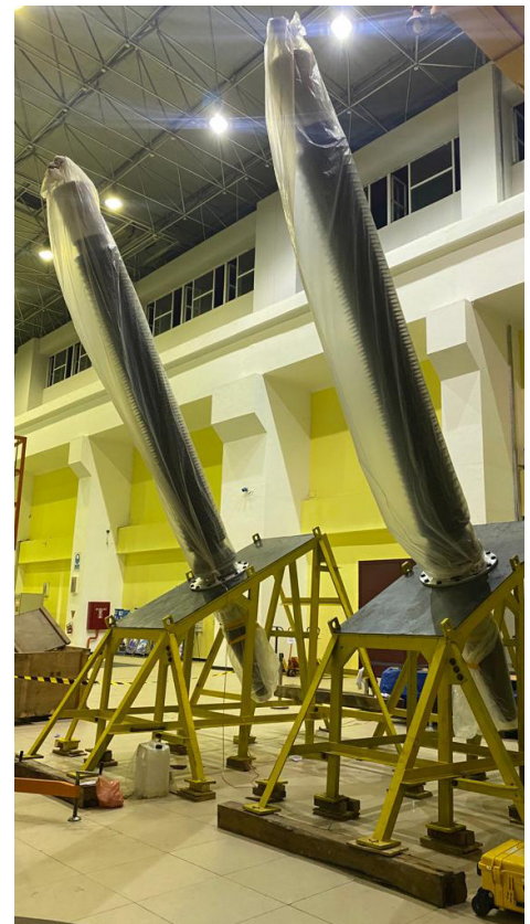
▶▶ TRANSFORMER BUSHING - PLTA Asahan - 1
