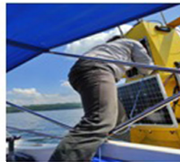
Instalasi Wave Buoy Project PLTS Terapung Cirata
